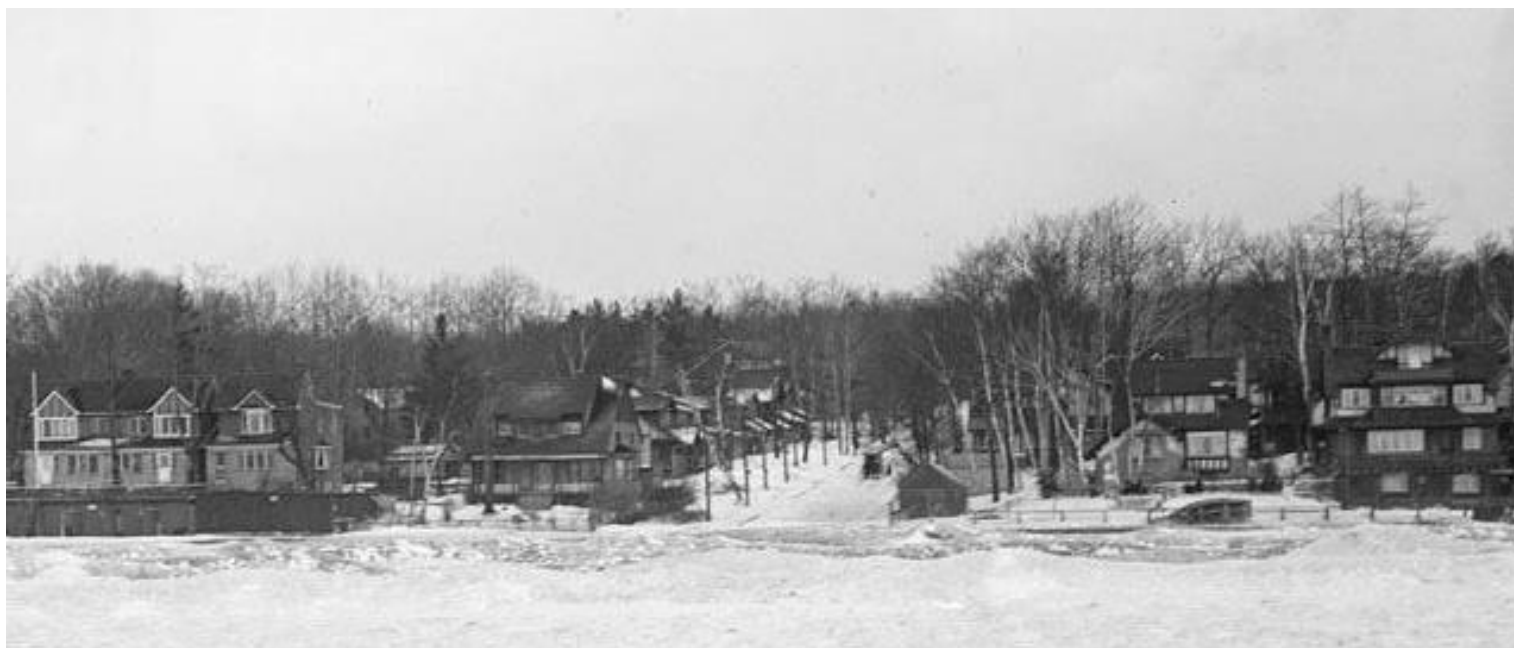
Detail from "Looking Up Silver Birch," 7 March 1924 [CTA, Series 372, Sub-series 3, Item 508] This view, from the frozen lake, shows lakefront houses both west and east of the street.
